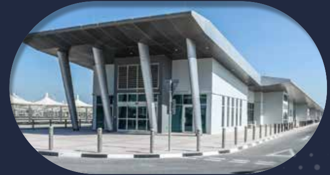
AIRPORT STAFF ACCESS CONTROL FACILITY (ASACF)
