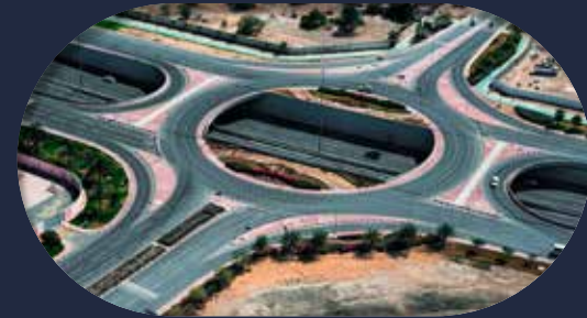
RAS ABU ABBOUD TUNNEL
