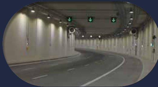
MALL OF QATAR TUNNEL
