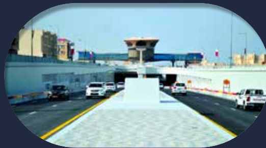
AL WAKRAH TUNNEL
